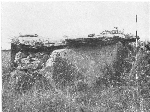
5. Commons North (Cl. 65) From North-West
