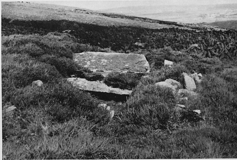
1. Sralagagh (Ma. 10) Roof of gallery from West
