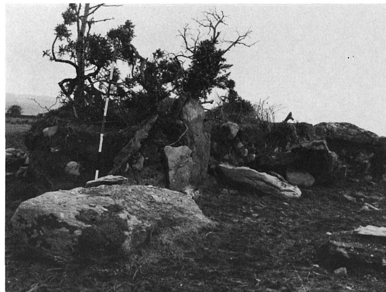
2. Carrownedan (Sl. 91) during course of demolition, from West.
