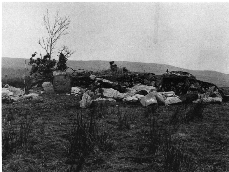
1. Carrownedan (Sl. 91) during course of demolition, from South.
